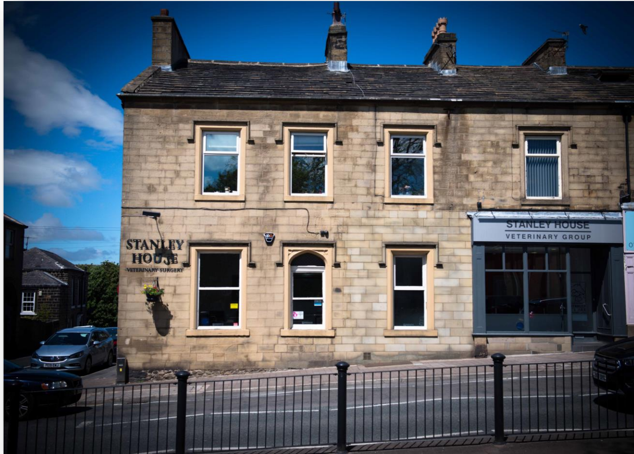
Stanley House Veterinary Group Exterior
